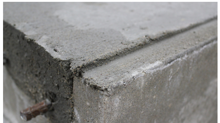
One Tool Strikes Off and Creates Slope to Drain
