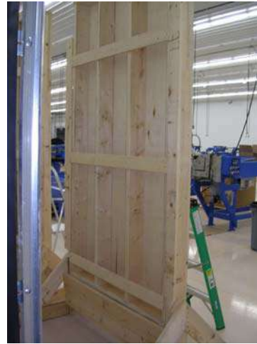
Figure 2: Rear view of frame construction
