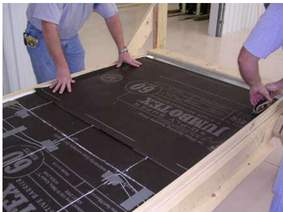
Figure 12: Installation of second paper layer
