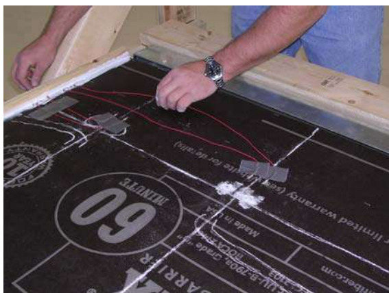
Figure 14: Affixing sensor wires
