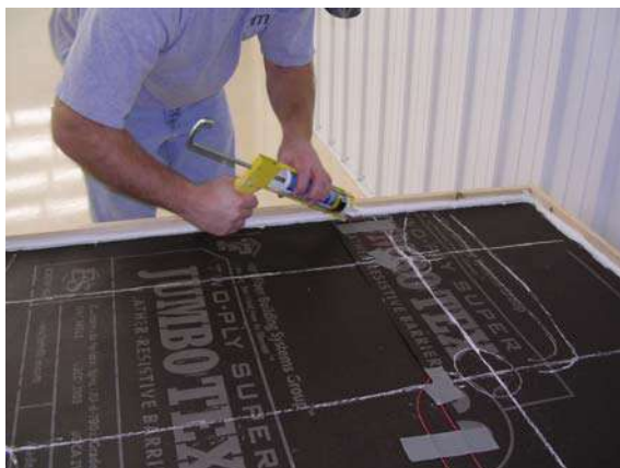
Figure 16: Sealing P2 edge
