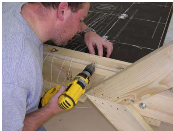
Figure 13: Drilling sensor wire guide holes
