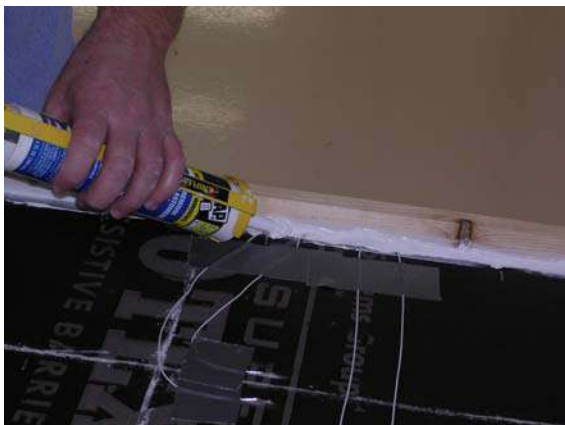
Figure 10: Sealing paper edge
