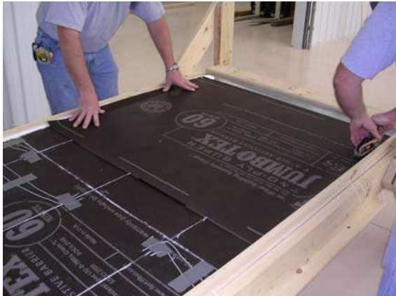
Figure 12: Installation of second paper layer
