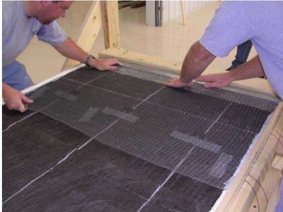
Figures 24: Installation of metal lath, Panel A
