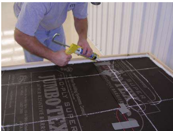
Figure 16: Sealing P2 edge
