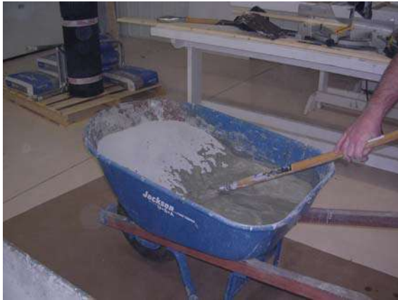
Figure 34: Mortar preparation
