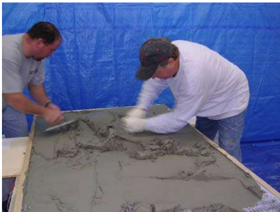
Figure 36: Mortar application
