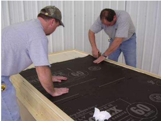
Figure 6: Construction paper placement
