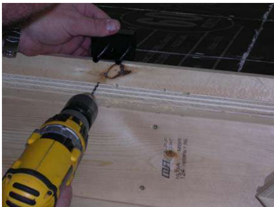
Figure 8: Sensor wire guide hole placement
