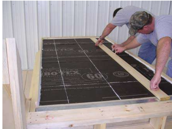
Figure 7: Marking grid pattern
