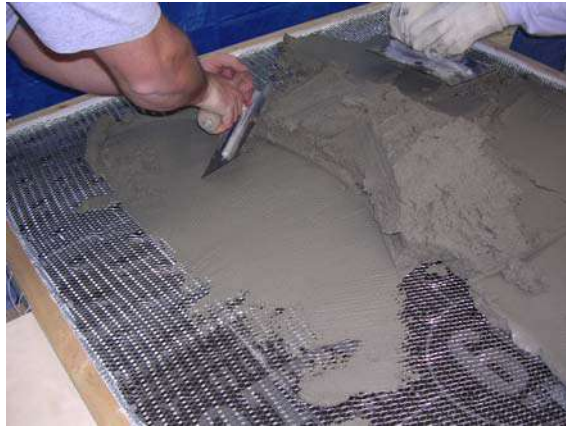
Figure 35: Mortar application
