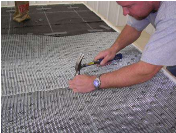
Figure 26: Installation of metal lath
