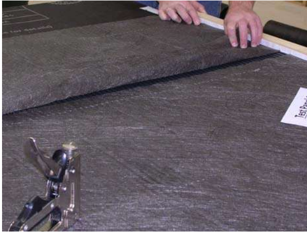
Figure 11: Installing Sure Cavity (SC 5032)
