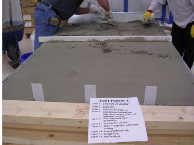
Figure 31: Applying Scratch Coat
