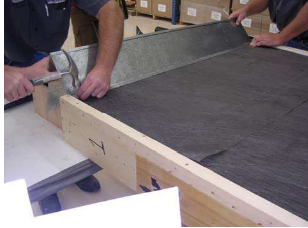
Figure 12: Installing Water Trough
