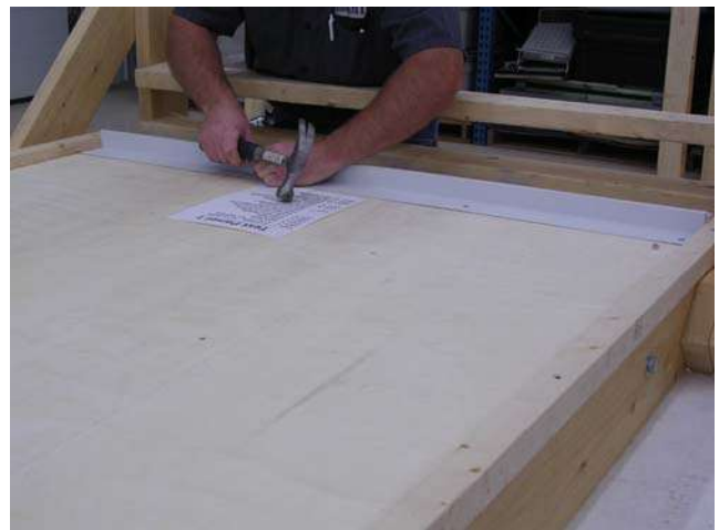
Figure 4: Installing Drip Plate
