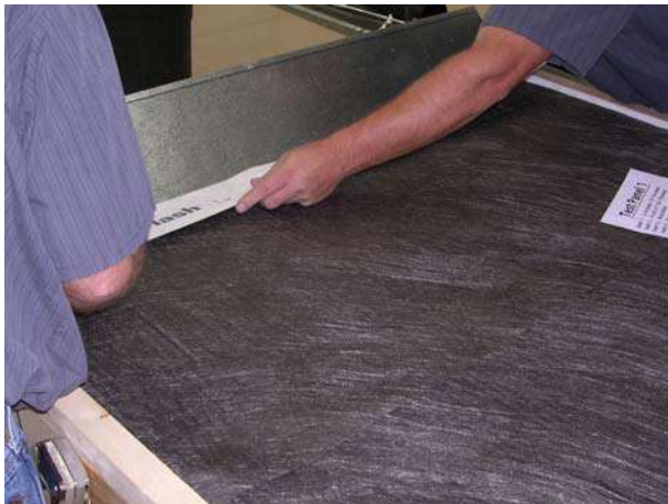
Figure 13: Installing Watertight Flashing
