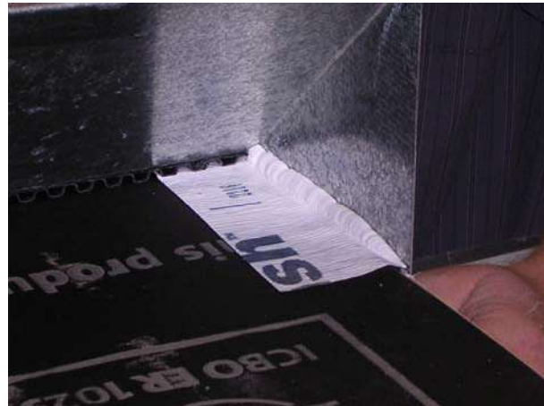
Figure 14: Caulking Edge of Trough
