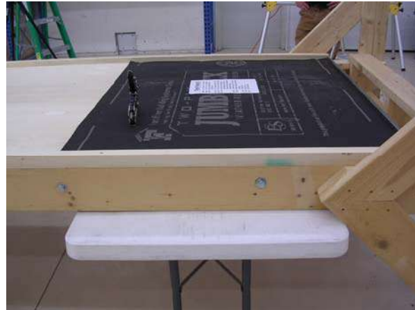
Figure 21: Installing Layers of Construction Paper
