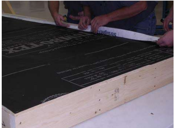
Figure 8: Applying Flashing to Perimeter
