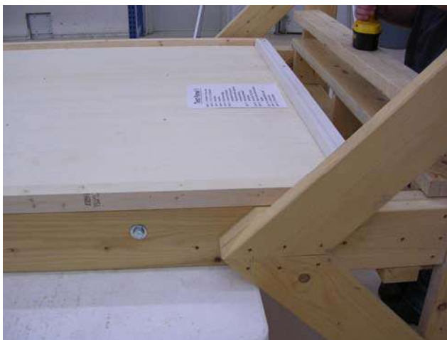
Figure 3: Installing Brick Mold
