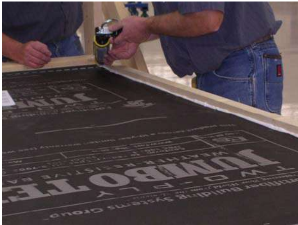
Figure 22: Caulking Perimeter
