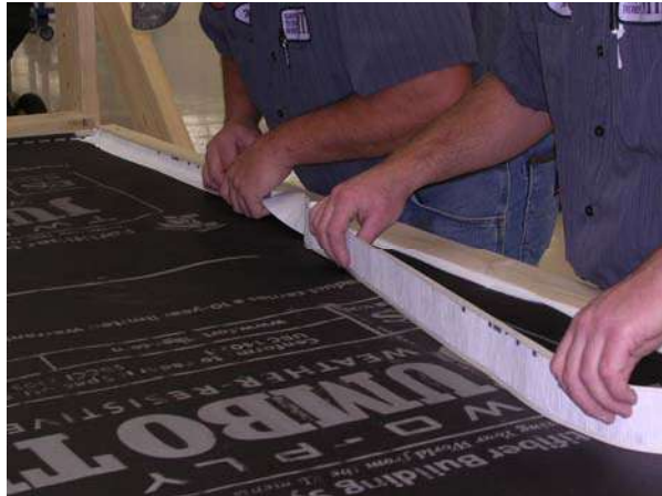
Figure 23: Applying Flashing to Perimeter
