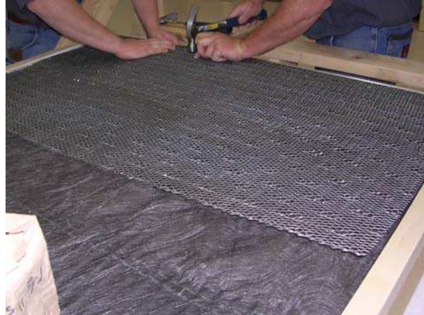
Figure 27: Installing Metal Lath
