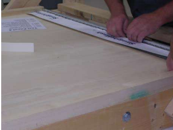
Figure 20: Installing Flashing
