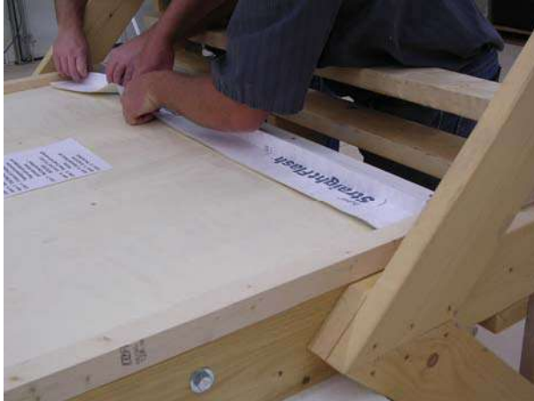
Figure 5: Installing Drip Plate Flashing
