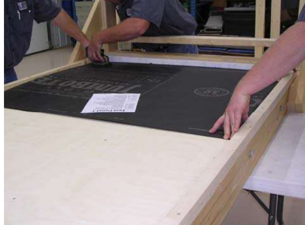
Figure 6: Installing Layers of Construction Paper
