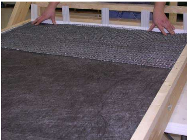
Figure 15: Installing Metal Lath
