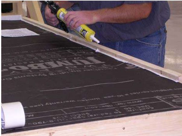
Figure 7: Caulking Perimeter
