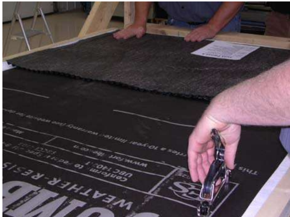
Figure 25: Installing 10mm Sure Cavity (SC2532)
