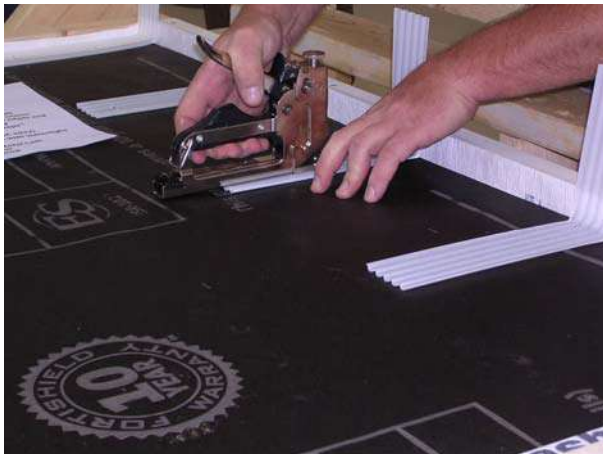
Figure 9: Installing Weeps
