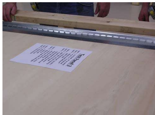
Figure 19: Installing L & R Weep Screed
