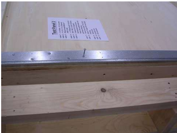
Figure 18: Installing Weep Screed Deflector
