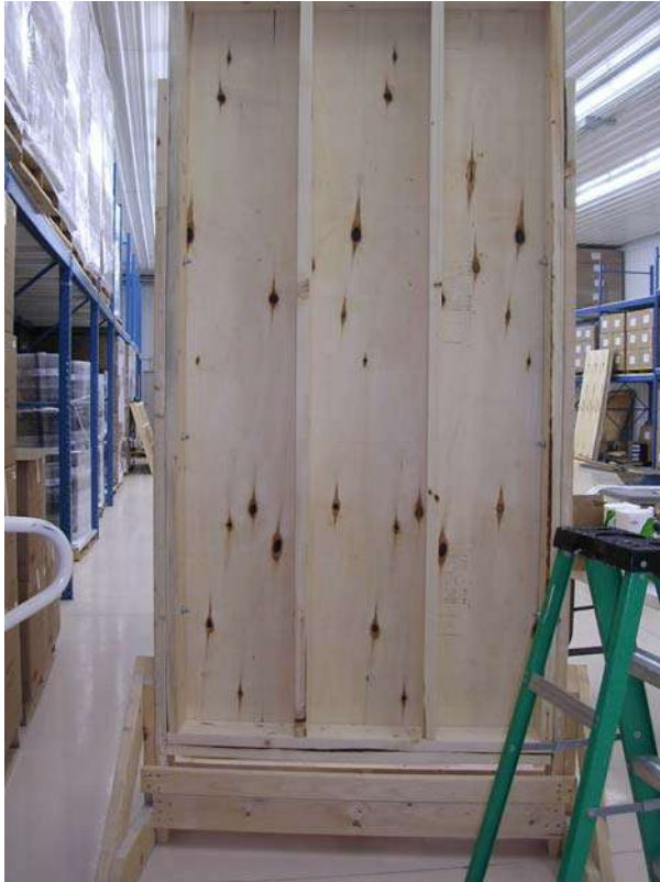
Figure 1: Back of Test Panels
