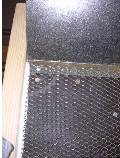
Wall A with Metal Lathe
