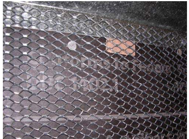
Spacers in Trough between paper and metal lathe
