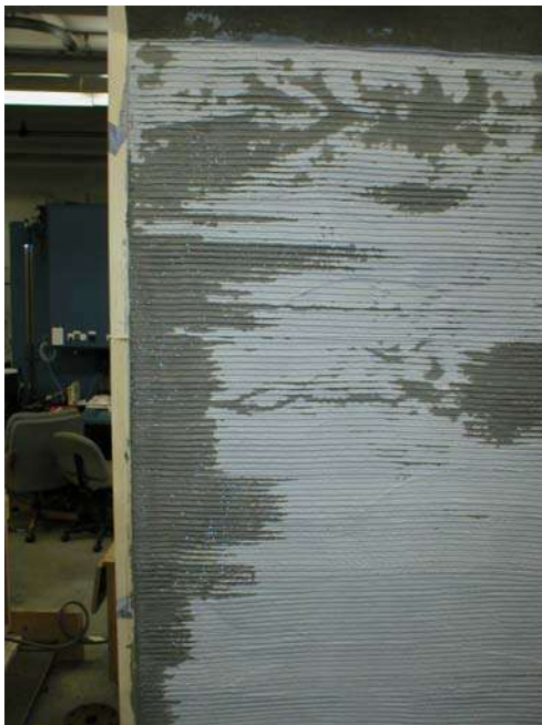
Wall A first test
