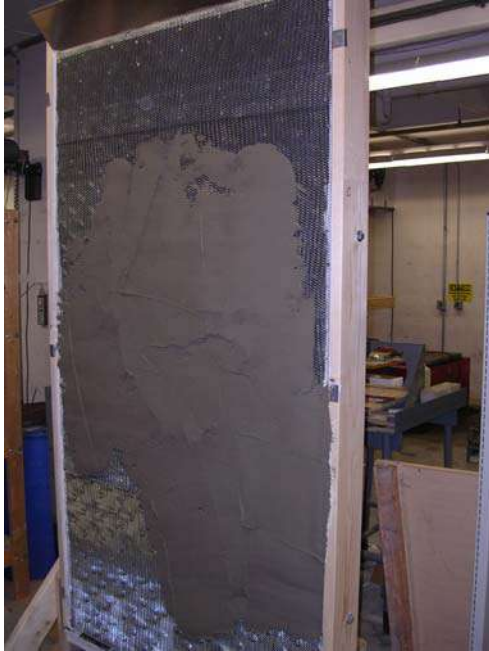
Application of Scratch Coat
