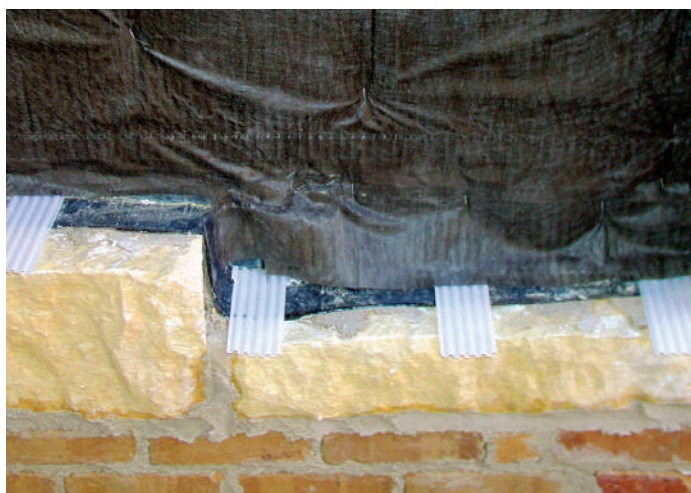
Wall Opening Weeps with Sure Cavity® on natural stone
