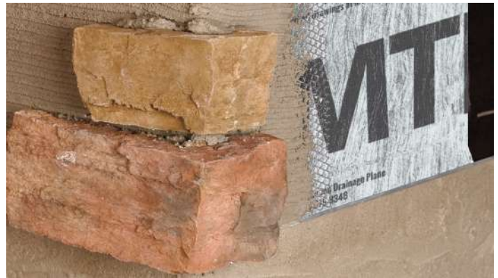
Thin Stone with Sure Cavity® rainscreen drainage plane
