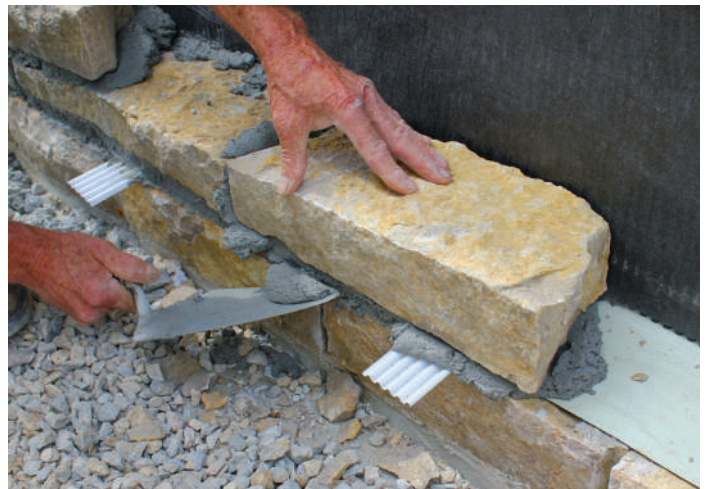
Stone Cavity Weep™ with Sure Cavity® on natural stone
