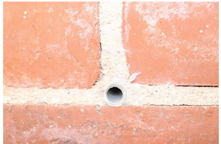
MTI Retrofit Weep™ used in a brick retrofit application
