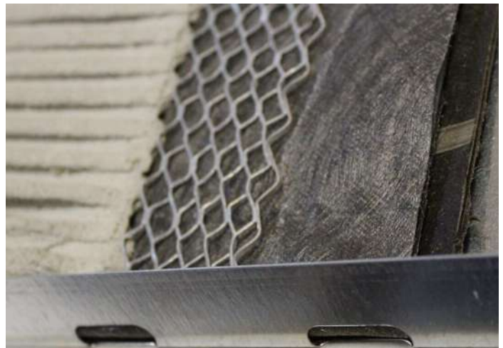
The WRB, rainscreen drainage plane, self furring lath, and scratch coat all fit inside the lip of the L & R Weep Scream™
