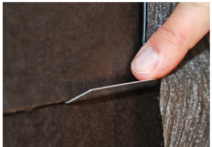
Moisture Diverter™ sloped-to-drain and integrated with WRB
