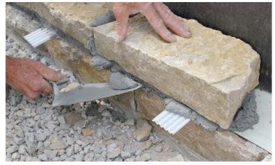
Stone Cavity Weep forms the bottom of the bed joint mortar
