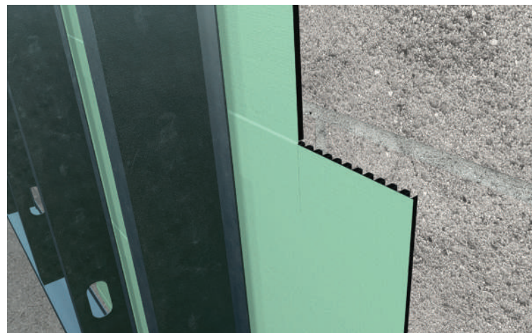
Perforated Control Cavity installed on interior of block wall
