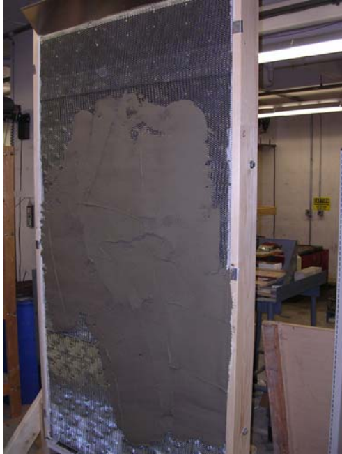
Application of Scratch Coat
