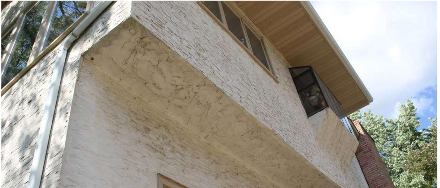
Figure 1: When stucco changes planes without a plan for drainage you get a stucco bucket. Buckets hold water - stucco wrapped soffits will too.
