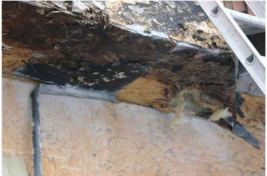
Figure 2: A “stucco bucket” on this stuccoed cantilever resulted in the wall kicking the bucket, so to speak. Water had nowhere to drain and eventually overwhelmed the WRB, rotting the framing beneath.
